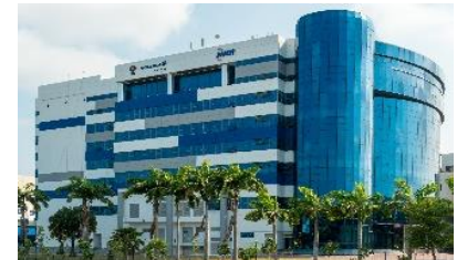
10 Changi South Lane
