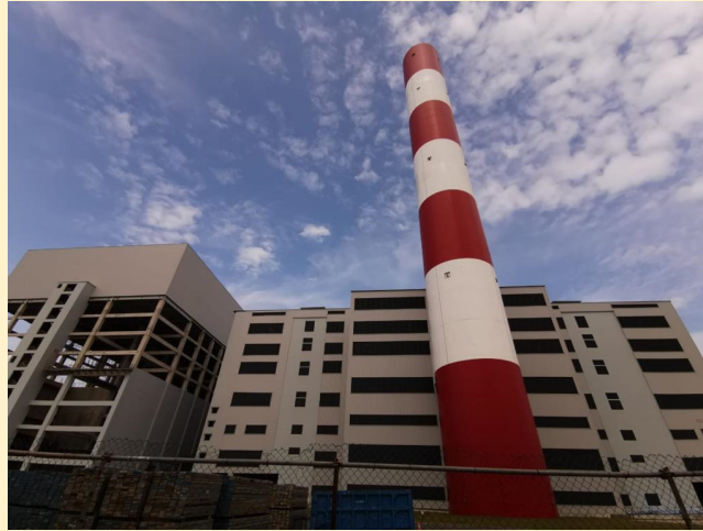
Ongoing construction of TuasOne WTE Plant, Singapore
