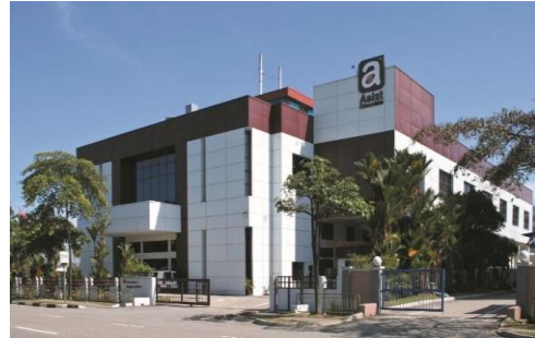
26 Tuas Avenue 7, Singapore
