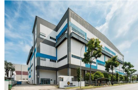
8 Tuas Avenue 20, Singapore
