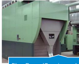
Blow Room (Opening and Transporting of cotton)
