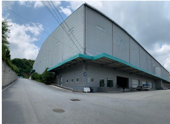
Mapletree Logistics Centre-Hobeob 2, South Korea
