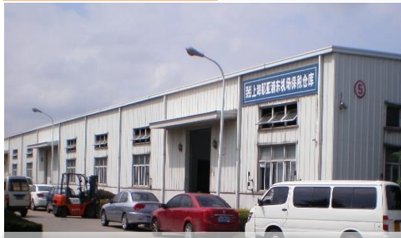
Ouluo Logistics Centre before redevelopment
