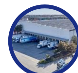
27-43 Toll Drive, Altona North
