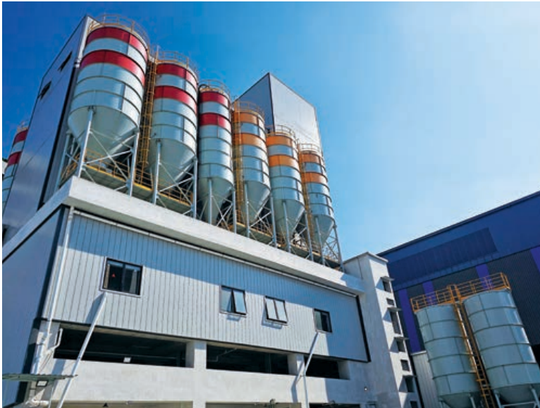
TMS Jurong Port batching plant
