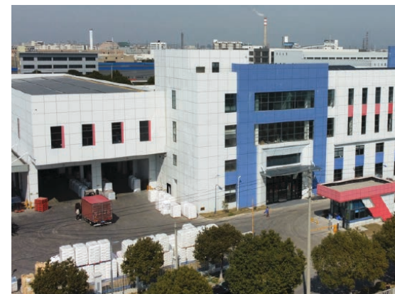
New R&P factory in Kunshan, Jiangsu China
