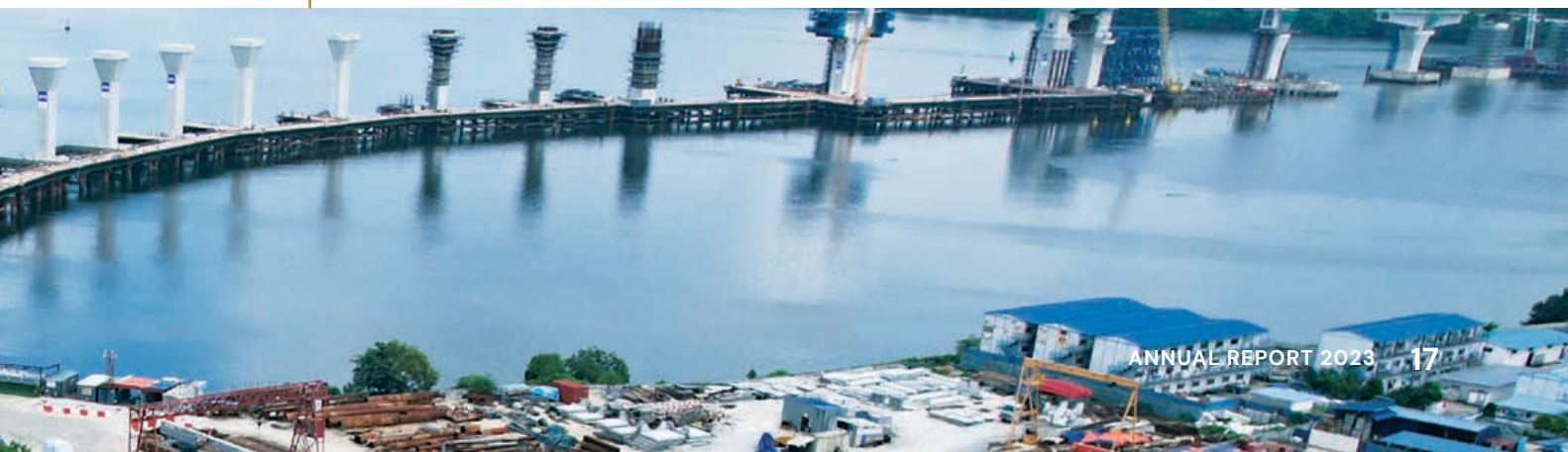
JB-SG RTS Link Marine Viaduct project
