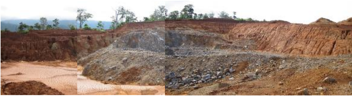
Figure 12-2 Pit Slopes at Buleleng
