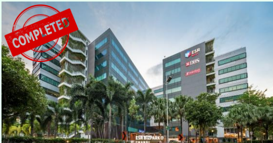
Asset Enhancement: ESR BizPark @ Changi (Business Park)
