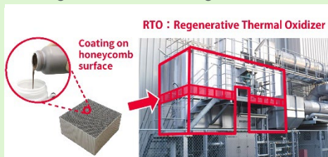
Environmental load reduction solutions: Heat-resistant ceramic catalyst material used in exhaust gas treatment at factories
