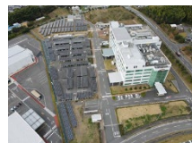
Carport-type solar power generation facility (Ise Murata Manufacturing)
