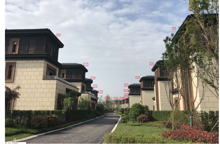
Villas : External Building
