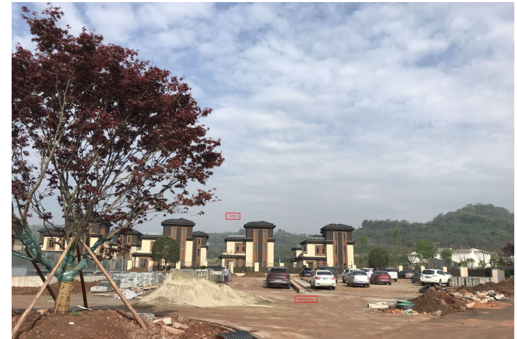
Villas : External Building
