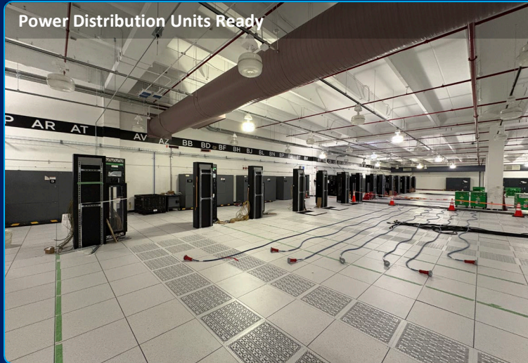
Raised Access Floor Replaced
