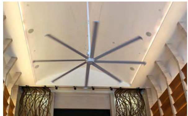
High Volume Low Speed Fan for up to 30% energy savings
