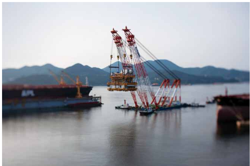
WHRUs being lifted onto FPSO, Angola
