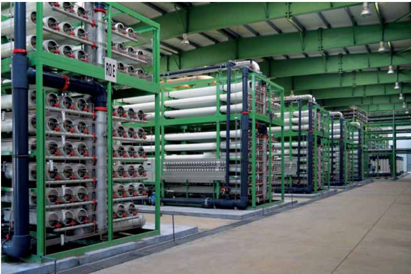
Wastewater recycling plant at Asia Symbol pulp & paper mill, China
