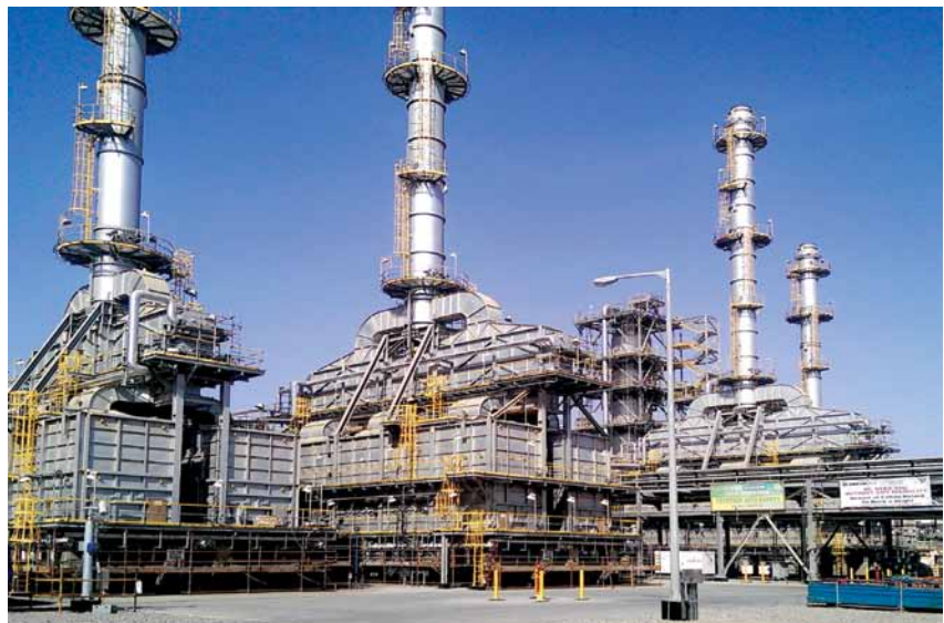
Reactor feed heaters, Saudi Arabia
