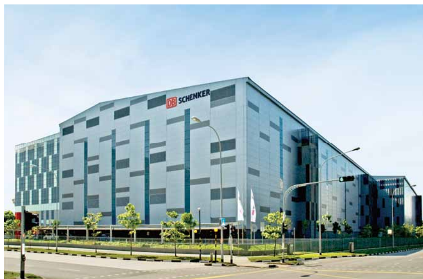
DB Schenker Shared Logistics Center 3 (Tampines LogisPark), Singapore
