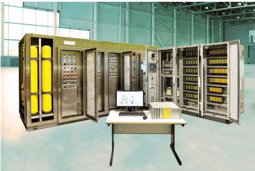
Smart wellhead shutdown systems, Saudi Arabia
