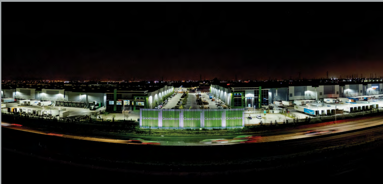
Goodman Commerce Center Eastvale, Los Angeles, USA.
