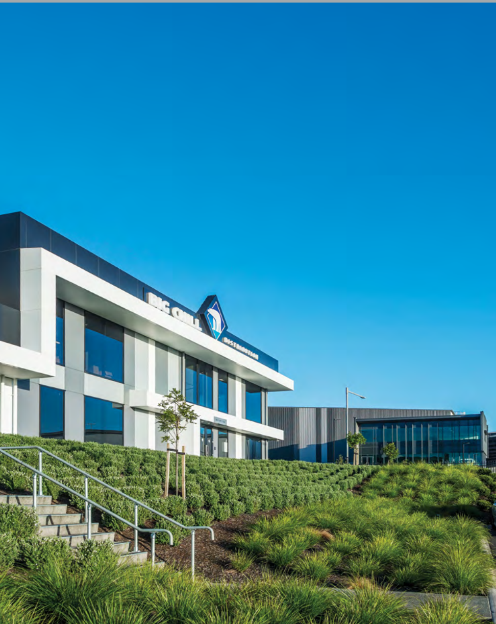
Highbrook Business Park, Auckland, New Zealand.
