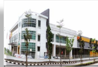
Quill Building 8 - DHL (XPJ)
