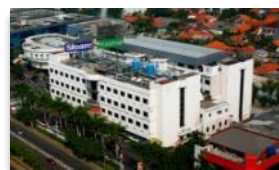
Siloam Hospitals Kebon Jeruk
