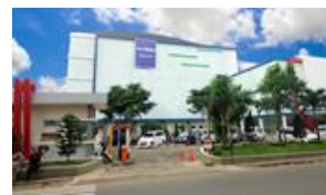
Siloam Hospitals Purwakarta
