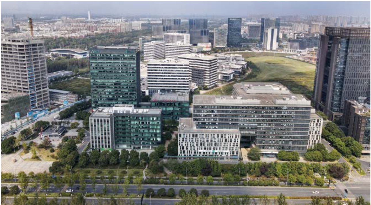
Singapore-Hangzhou Science & Technology Park Phase I
