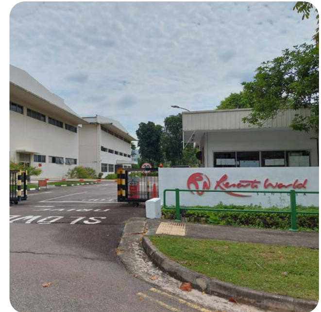
RWS warehouse in Pandan Garden powered by solar energy
