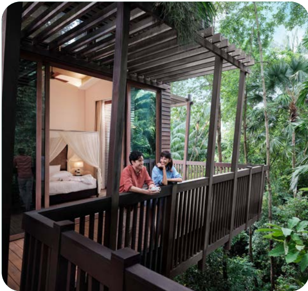
Equarius TreeTop Lofts, surrounded by preserved secondary forest that provides a natural cooling effect
