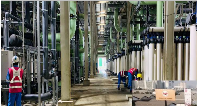
TSEPC project: Replacement of UF Membranes at Tuas South Desalination Plant, Singapore.
