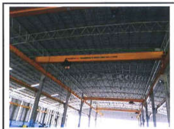
OVERHEAD CRANE 5 TONS SHOP 1 - OC-056
