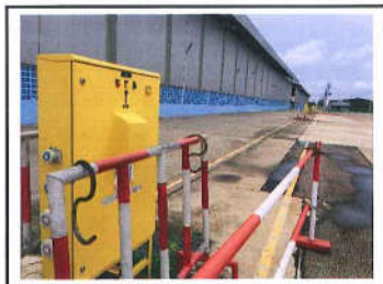
MDB WATER PROOF TYPE-3-PHASE 300A/100A/30A/16A
