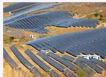
山地光伏 Mountain Photovoltaic
