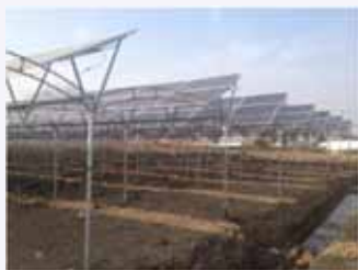
光伏大棚 Photovoltaic Greenhouse
