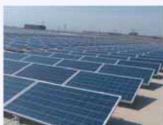
光伏屋顶 Photovoltaic Roof
