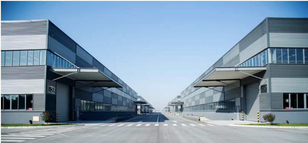
Changshu Fervent Industrial Park, Jiangsu
