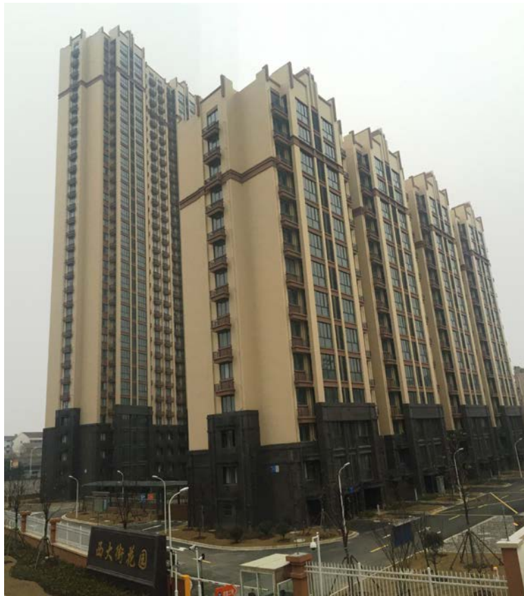
Residential Build-and-Transfer Project, Jiangyin
