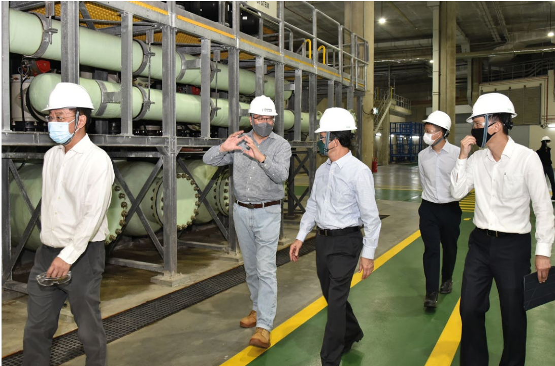
KIFM Directors and Management visited the Keppel Marina East Desalination Plant, prior to the signing of a non-binding term sheet with sponsor Keppel Infrastructure in June 2022 to acquire a 100% economic interest in the plant.
