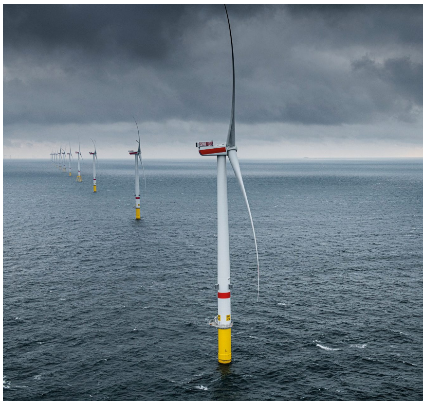
BKR2 has an operating capacity of approximately 465 MW and is located 59km off the coast of Lower Saxony in the North Sea, Germany.
