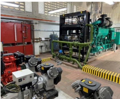
Replacement of 6.6V and 400V Diesel Generators at 9 Catchment and Waterways Installations.
