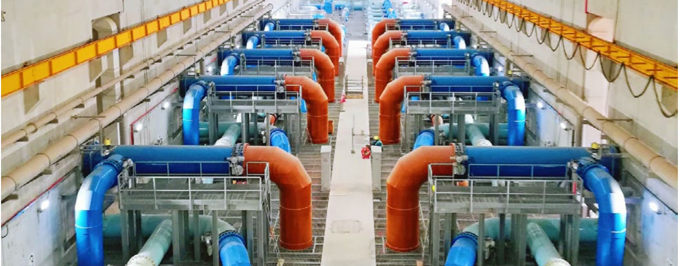
Process upgrading at Choa Chu Kang Waterworks - Ozone and Biologically Activated Carbon Facilities.
