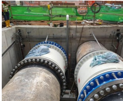
Electrical, Instrumentation, Control and Automation Works for Murnane project at Murnane Reservoir.
