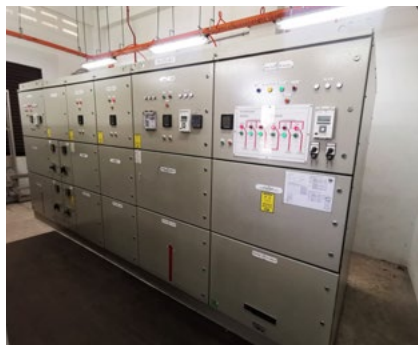
Expansion of Plant Power Supply at Jurong Water Reclamation Plant.
