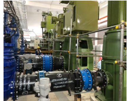
Replacement of pumpsets at Kranji and Tengeh Pumping Station.
