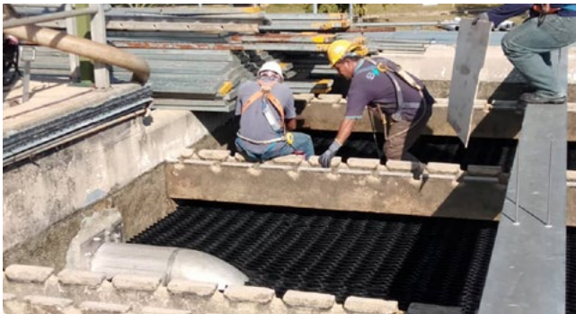
Maintenance of Electrical Motors and Actuators at Johor River Waterworks.
