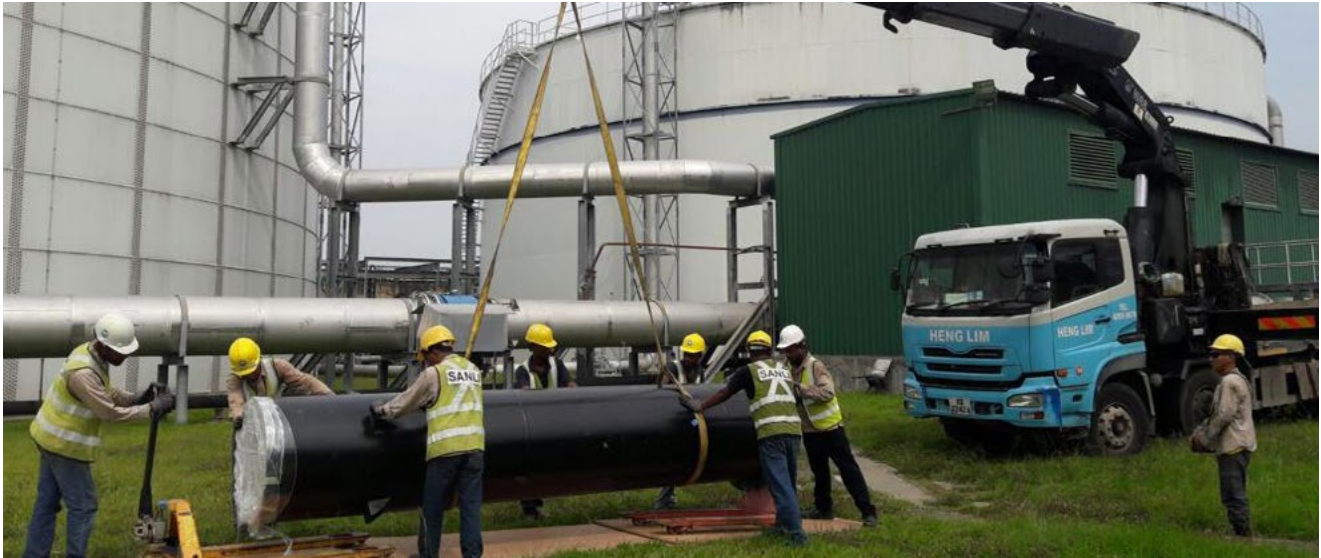
Overhaul of Pumps in Catchment & Waterways.
