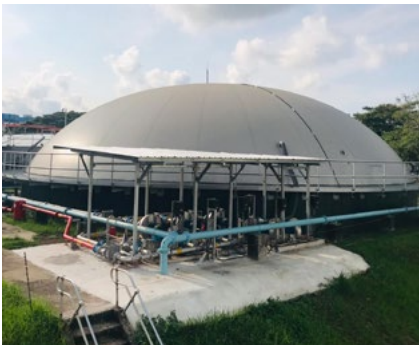
Replacement of Mechanical and Electrical Equipment at Ulu Pandan Water Reclamation Plant.
