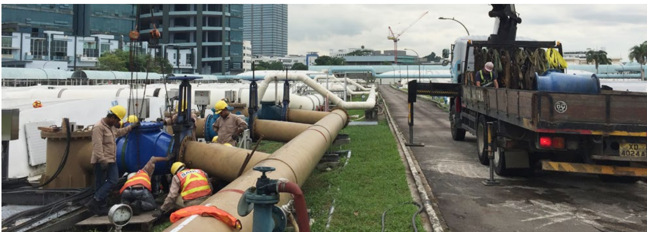
Servicing and Maintenance of Screening, Sludge, Grit and related equipment at various Water Reclamation Plants.
