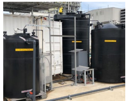
Design, Engineering, Manufacturing, Testing, Delivery and Erection & Commissioning of FO-RO Pilot Plant.
