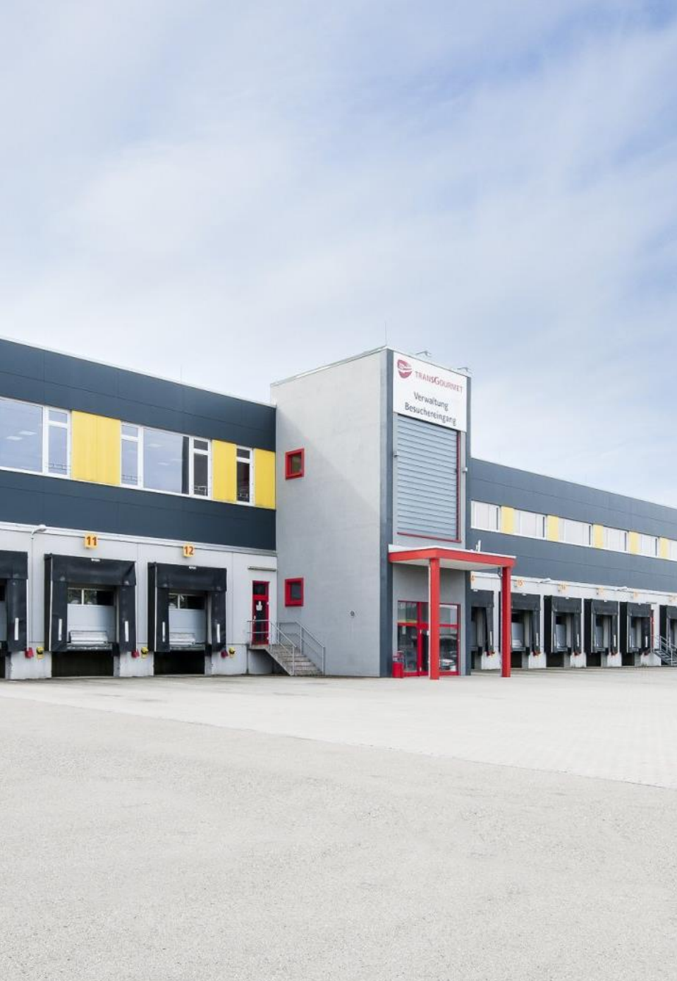
Transgourmet Facility, Ulm, Germany
