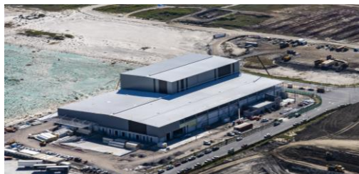
Corner Heron Drive and Curlew Street, Port of Brisbane, QLD (under construction)
