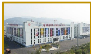
Fu Heng Warehouse
