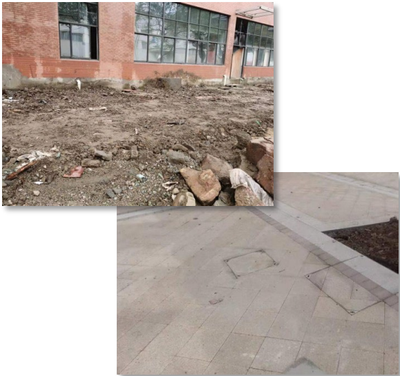
Images on the construction on-site
