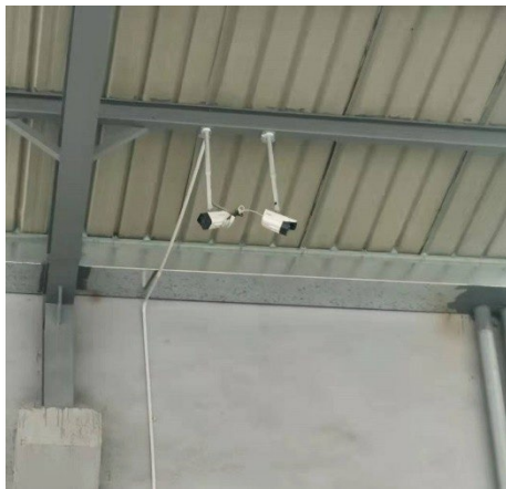
An example of new CCTV equipment installed in Phase I and II of Hengde Logistics
