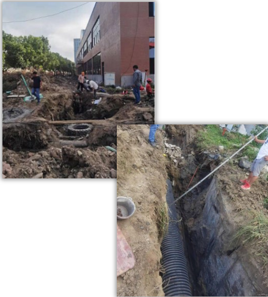
Images from the previous renovation
