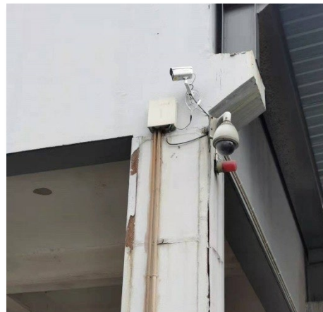
An example of new CCTV equipment installed in Phase I and II of Hengde Logistics
