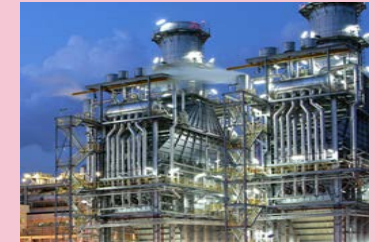
A top-tier gas-fired power plant in Singapore
