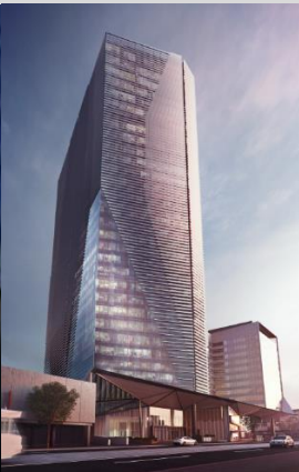
311 Spencer Street Melbourne (50% interest) -Under construction-
