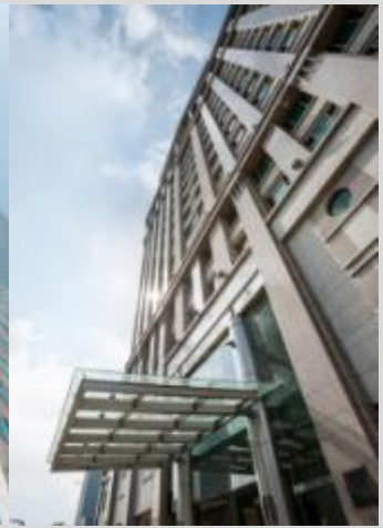
Bugis Junction Towers (100% interest)
