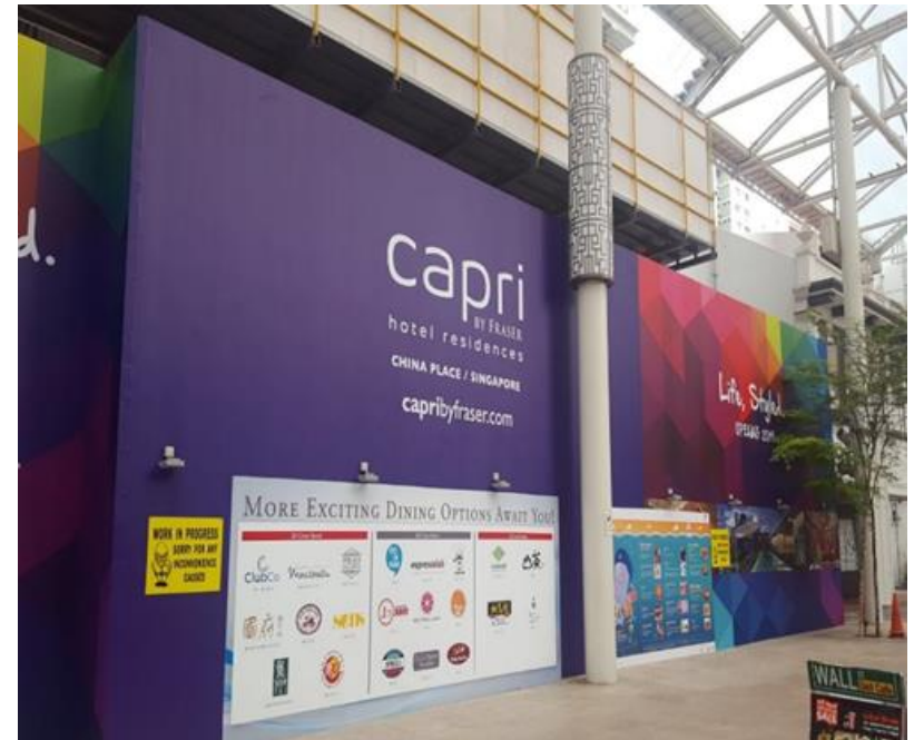
Construction hoarding along Nankin Mall
