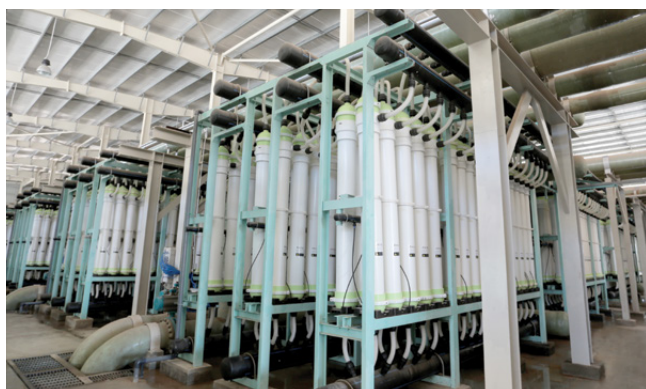
World's largest ultrafiltration pre-treatment installation, Magtaa Desalination Plant, Algeria
