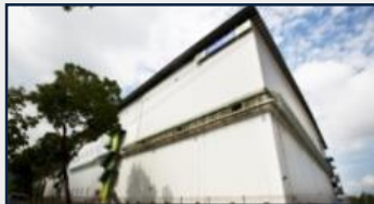
2 ALOG Cold Centre 2 Fishery Port Road
