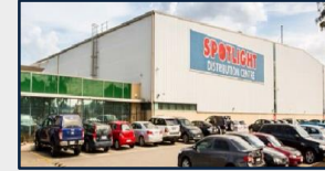
19 217 – 225 Boundary Road, Laverton North
