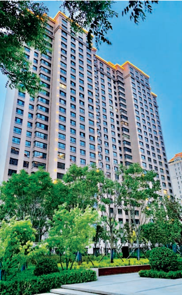
Tangshan Nanhu Eco-City project
