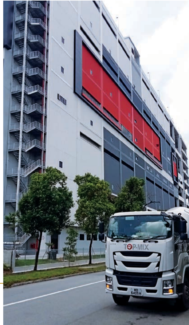
Pokka building at 4 Benoi Crescent
