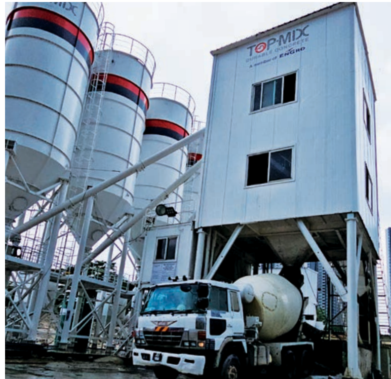
TMM batching plant
