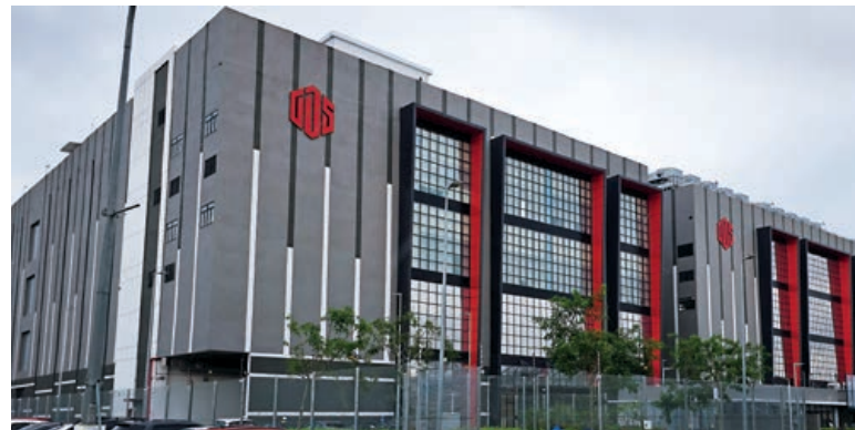
Data center owned by GDS at Johor, Malaysia
