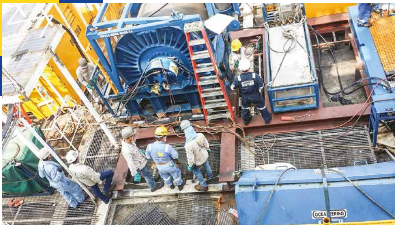
Above: Mobilisation of full Remotely Operated Vehicle (ROV) System.
