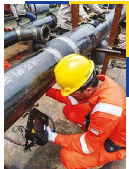
Above: Non-destructive testing conducts on fabricated pipe joints
