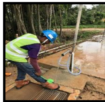
Washing of muddy water shoe using recycled water
