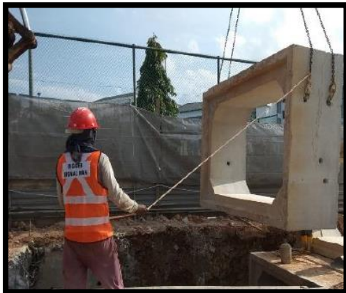
Usage of pre-cast to minimise rebar or concrete use
