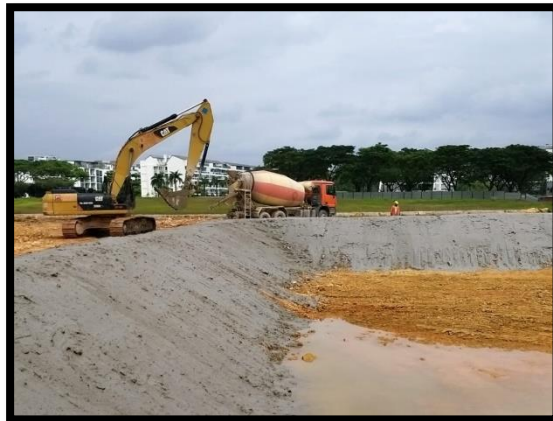
Use of sustainable material LSS for slope protection
