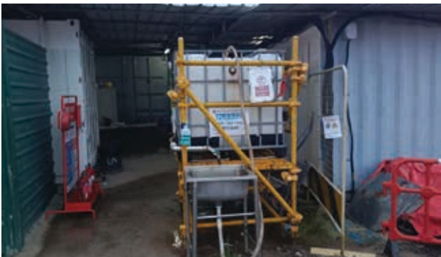
Re-Use of scaffold pipes to construct Water Tank Stand
