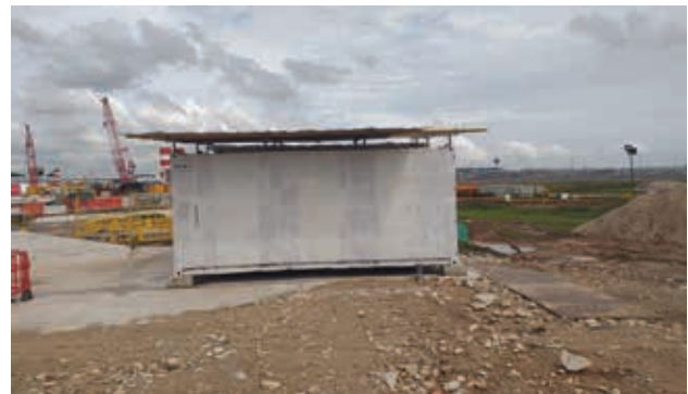
Re-Use of zinc sheets to construct Container Pitched Roof
