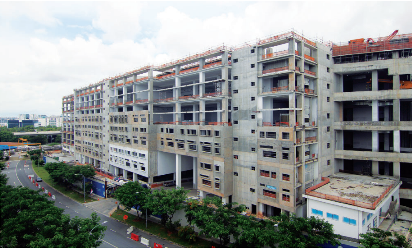
▲ Ongoing Project - Defu Industrial City
