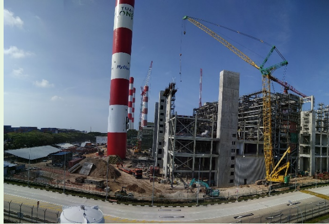
Ongoing construction of TuasOne WTE Plant, Singapore
