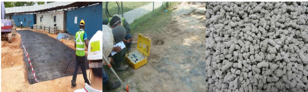
Temp Access Road
