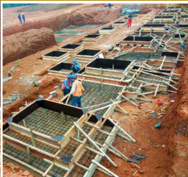
∧ pouring of concrete foundation
