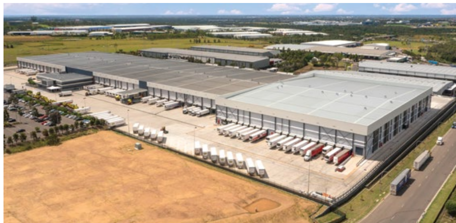
Coles Chilled Distribution Centre
