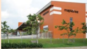
122 Mapletree Logistics Centre
