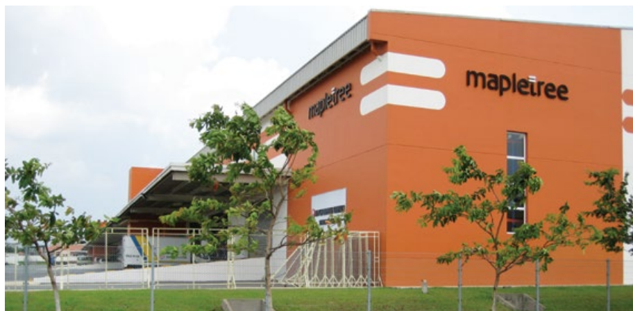
Mapletree Logistics Centre
