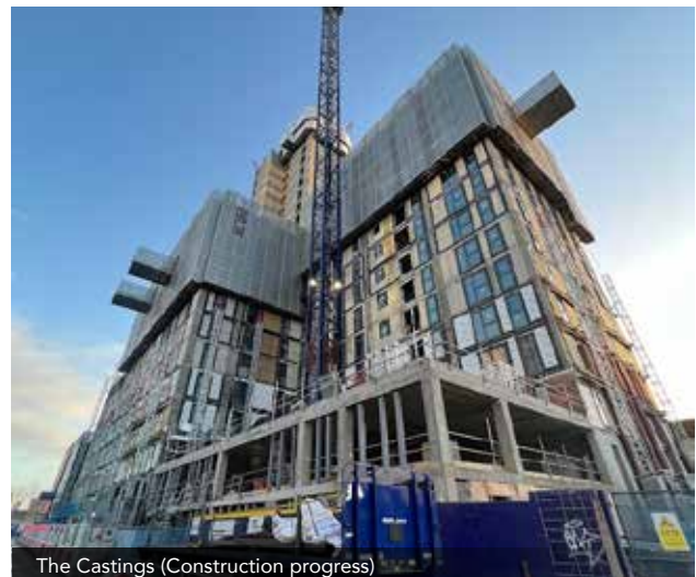
The Castings (Construction progress)
