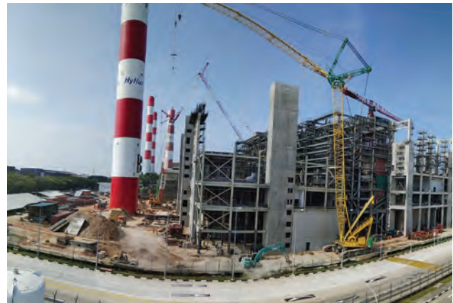
Ongoing construction of TuasOne WTE Plant
