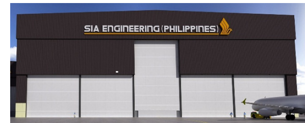
Hangar 3 2014 (under construction) 1 bay: widebody aircraft
