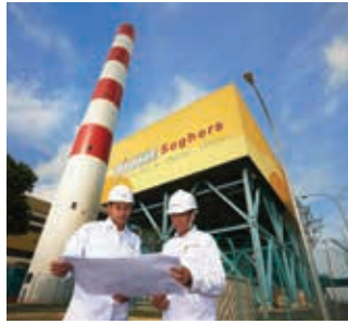
Tuas DBOO Plant
