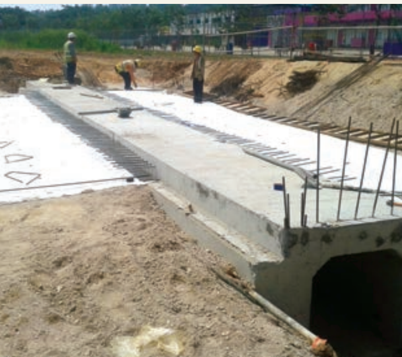
OKP is involved in the widening of Tanah Merah Coast Road.
