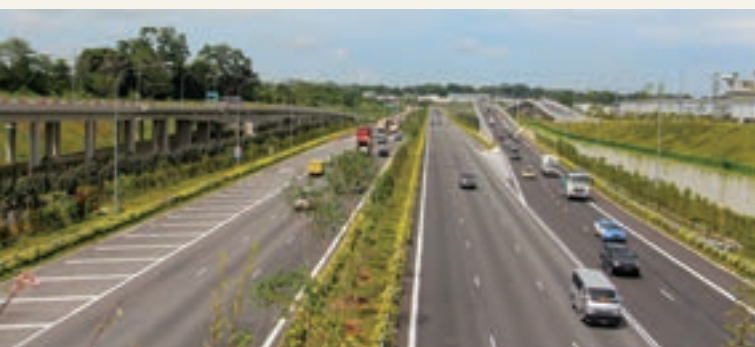
OKP has completed the design and build of interchange at TPE/Sengkang West Road/Seletar Aerospace Way in 2014.
