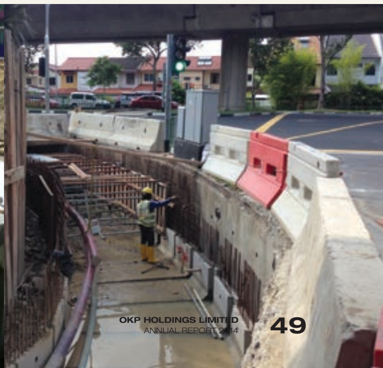
OKP has completed Improvement to roadside drains at Chai Chee Road/ New Upper Changi Road in 2014.
