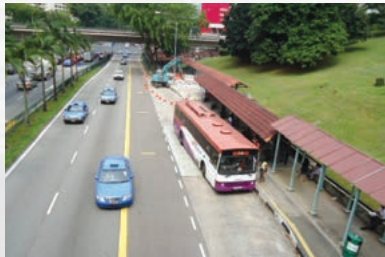
OKP is involved in ad hoc repairs and upgrading of roads, road-related facilities and road structure in Central Singapore.
