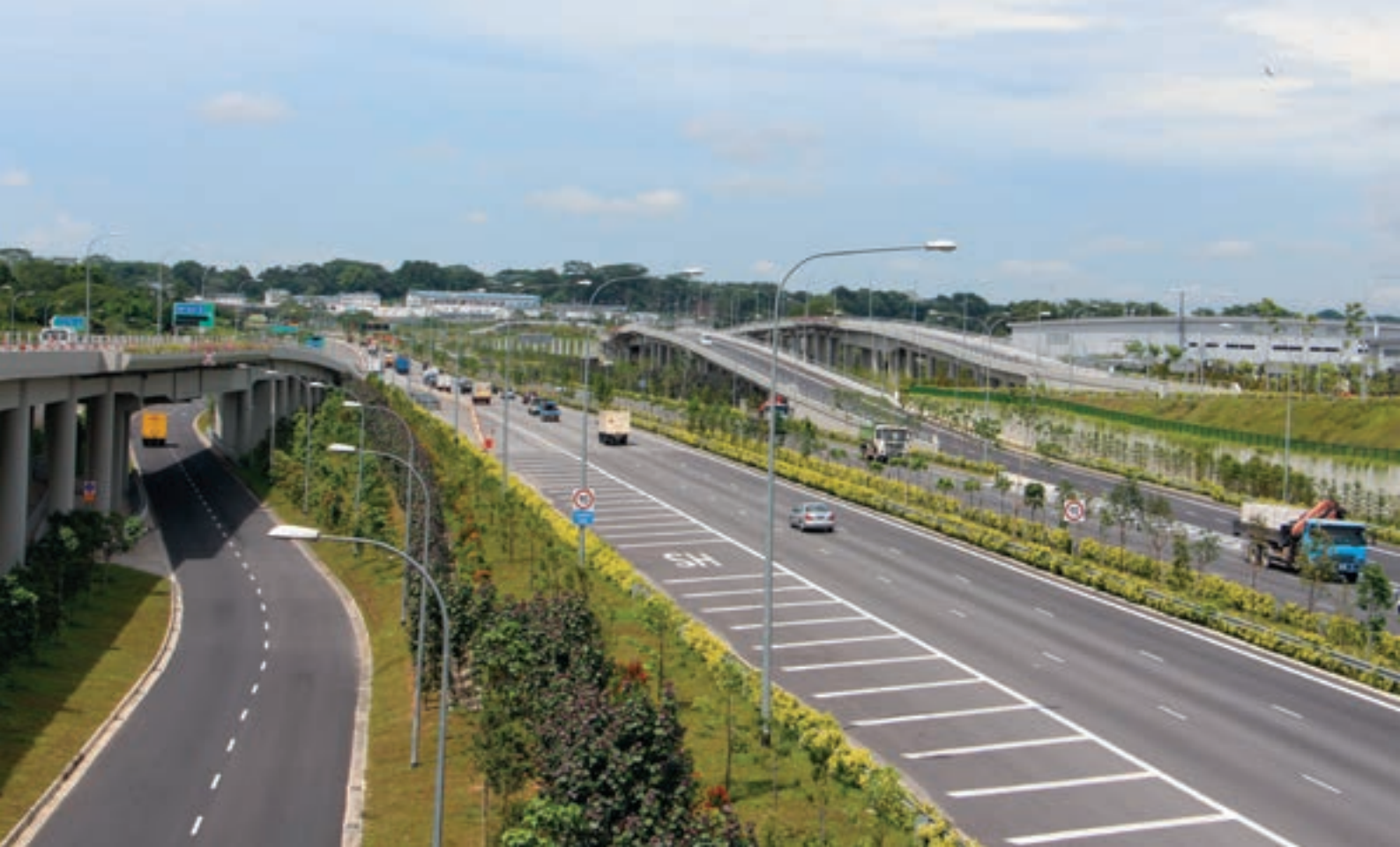
OKP has completed the design and build of interchange at TPE/Sengkang West Road/Seletar Aerospace Way in 2014.
