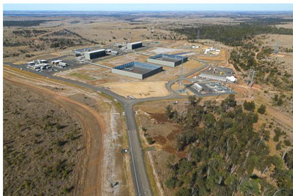
Eurombah Creek Gas Processing Facility
