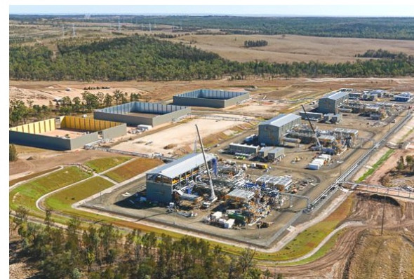
Combabula Gas Processing Facility
