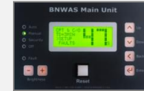
Bridge Navigational Watch Alarm System
