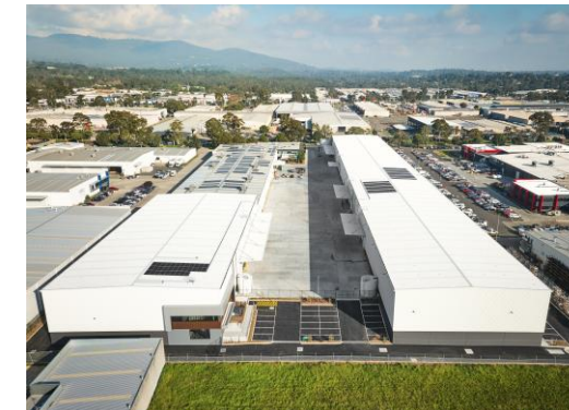
Australia | Kilsyth Solar Capacity: 300kW
